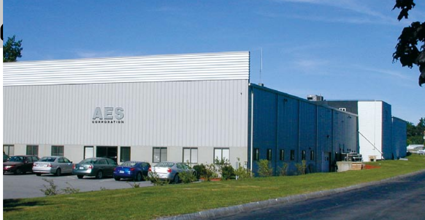
■ AES Corporation corporate office building
